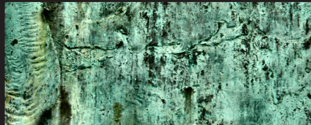
FIGURE 2 - OXIDATION OF A COMPRESSOR INTERNAL SURFACE
