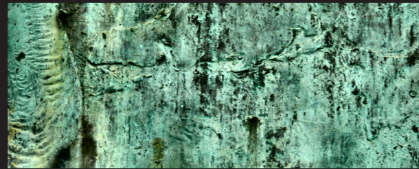
FIGURE 2 - OXIDATION OF A COMPRESSOR INTERNAL SURFACE
